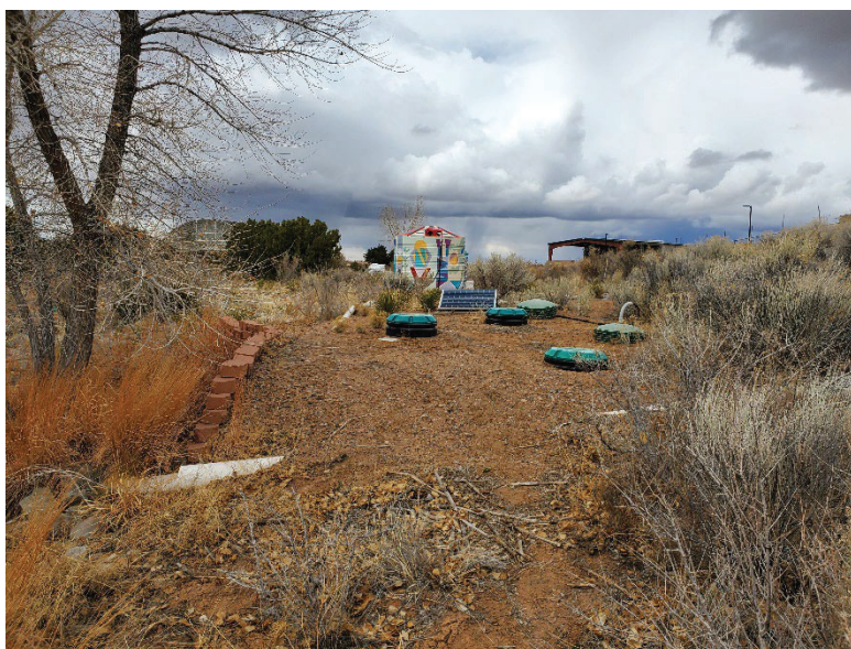
Figure 5. Existing rainwater tanks with below ground tanks in foreground (only shown are tanks access points).
