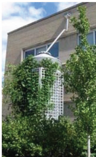
Figure 4. A tall building with a large metal cistern to collect stormwater runoff from the roof. From the Environmental Protection Agency.
